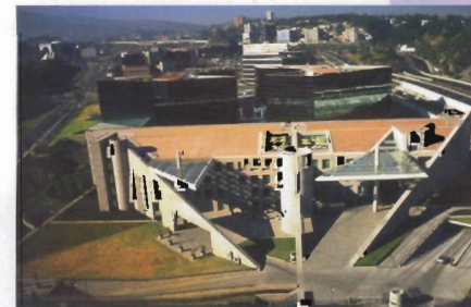
The Mexico City facility was built in two phases. The right side was completed in 1995 and the left side in 1997.
